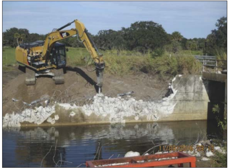
Figure 12. Demolition of the old control structure.
