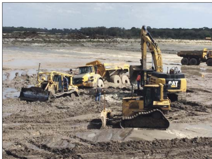
Figure 6. Contractor working in adverse conditions.
