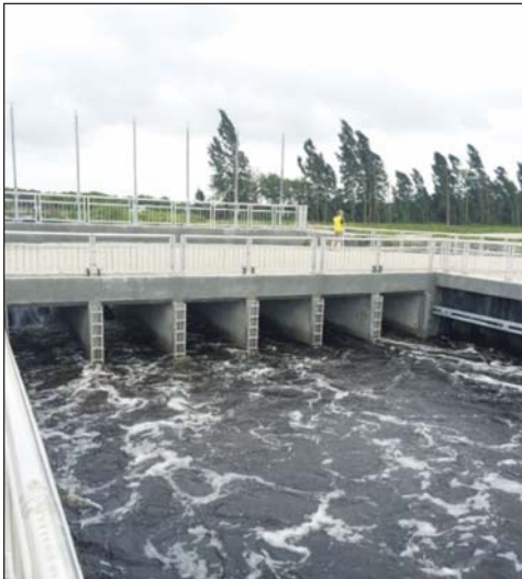
Figure 8. Looking upstream at Control Structure 1 during Tropical Storm Hermine.
