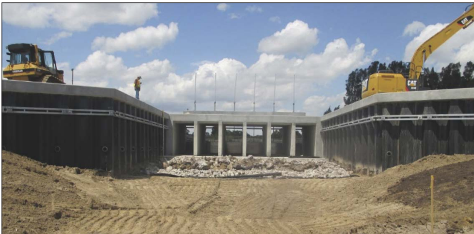
Figure 10. Construction of Control Structure 1.
