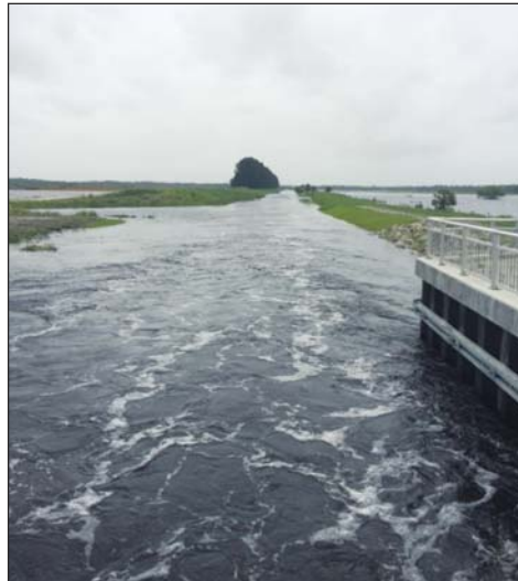
Figure 9. Cow Pen Slough looking downstream from Control Structure 1 during Tropical Storm Hermine.
